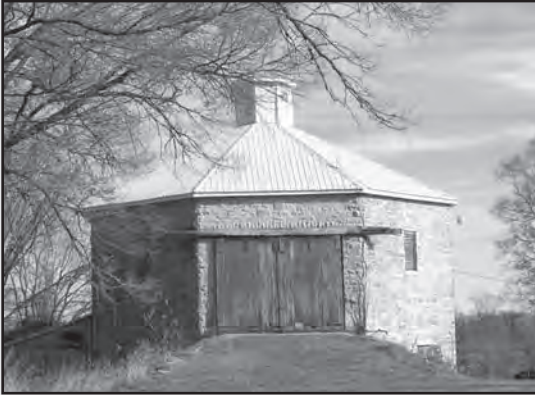
Octagonal stone barn in Clark County
