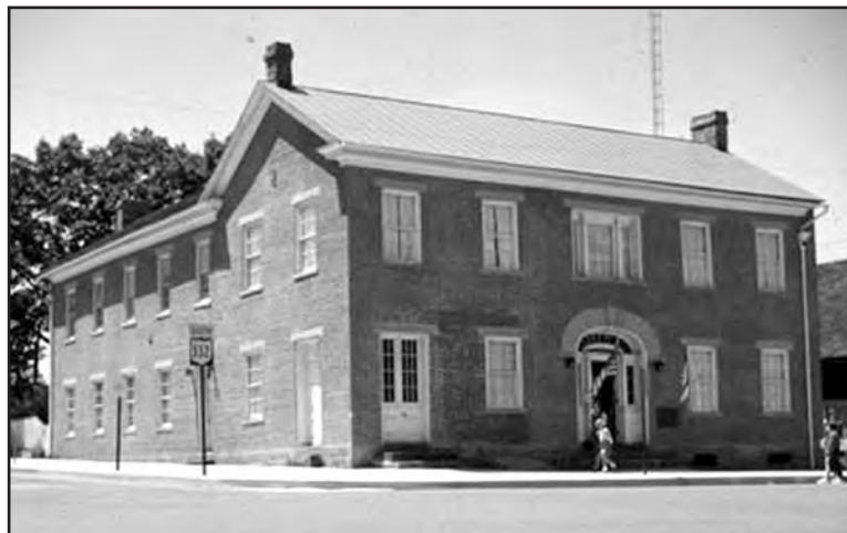
Image: Carroll County Historical Society website Mc Cook House in Carrollton, built in 1837 in the Federal Style. An I-House with chimneys built inside the end-walls and a large addition at the rear. Now a historic house museum operated by the Carroll County Historical Society.
