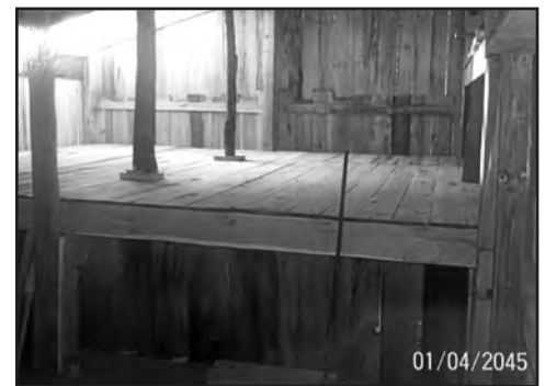
The 'Skellet effect.' The loft and walls repaired.
