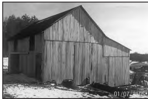
Canted queenposts with struts supporting purlins and the roof system.
