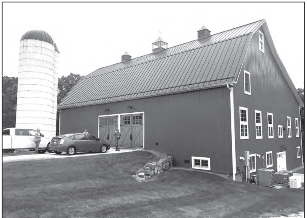
Repurposed barn that will be registration stop for the Friday barn tour.
