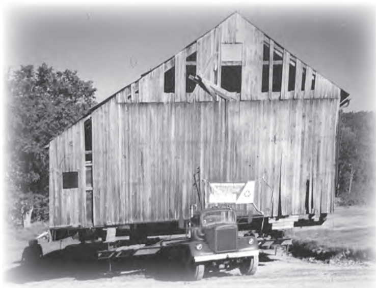
Sweitzer barn being moved on the farm.
