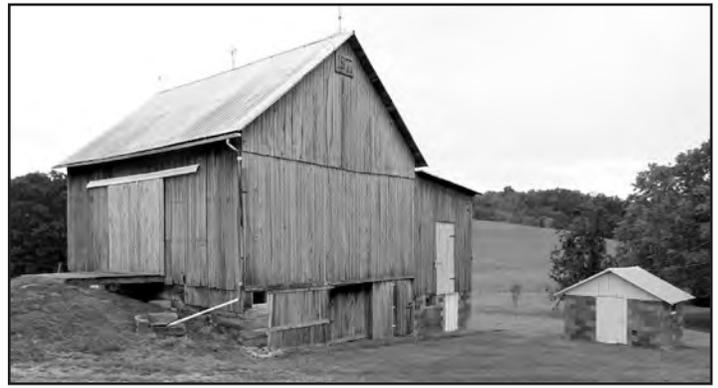
The new bridge built to the threshing floor takes the pressure of the earthen ramp off the restored sandstone bank wall below. Doors were replaced at the entry to the threshing floor and to the hay storage above the milking parlor with the clay block foundation at the far-right end of the barn. Fred installed the metal roof and lightning rods in the late 1940's and built the milking parlor and hay storage addition in 1948. Note the recently planted tree between the milkhouse and milking parlor.
