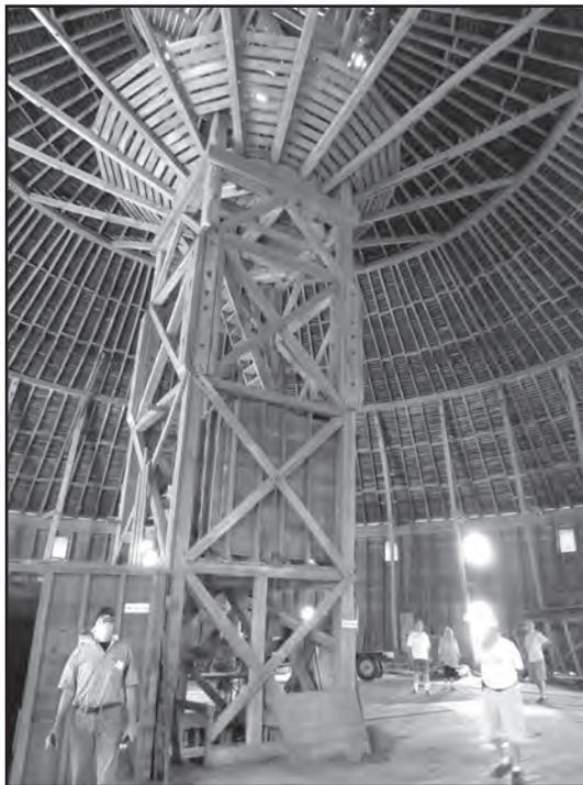
**Left: Chuck Bultman and Rudy Christian studying the center of the Littleton-Kingen Round Barn where a massive wooden tower once supported a wind driven system that provided water for the cows.**
