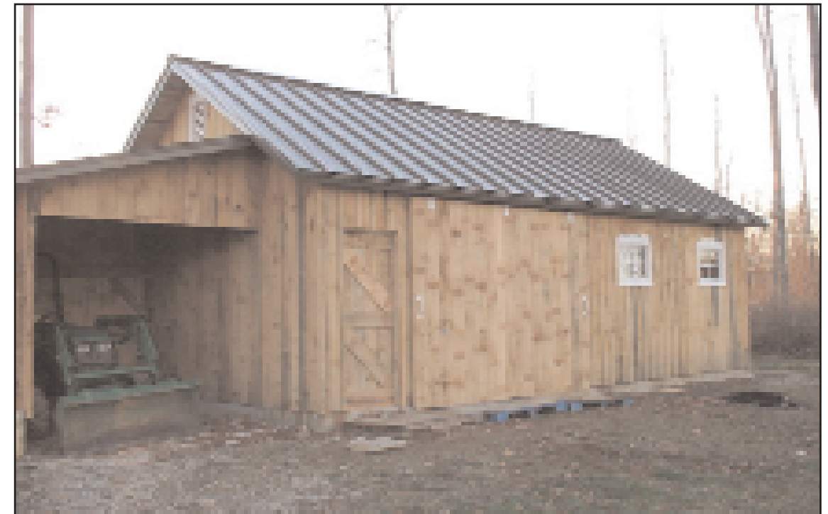
Above: This finished workshop was reconstructed from a Licking County barn and moved to its new home in Morrow County. It will be painted barn red with white trim. Below: The original Licking County barn was 20 by 30 feet with a shed addition on the back. Part of that shed was used to make a new shed for tractor storage.
