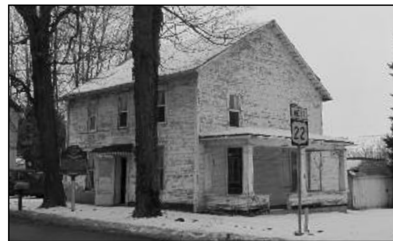
The Jacob Miller log tavern on Zane's Trace in Somerset. Logs cut in the early 1800s sprouted as seedlings between 1663 and 1715. The building was recently purchased by the Perry County Historical Society.
