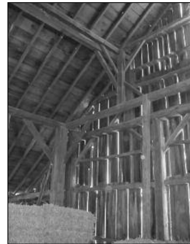
Above: Double framing in the Poorman barn. Right: Double posting of hewn timbers in the corner. Left: Marriage marks at the foot braces. Below: Door handles are cut in the shapes of moon phases: full, half, and crescent.
