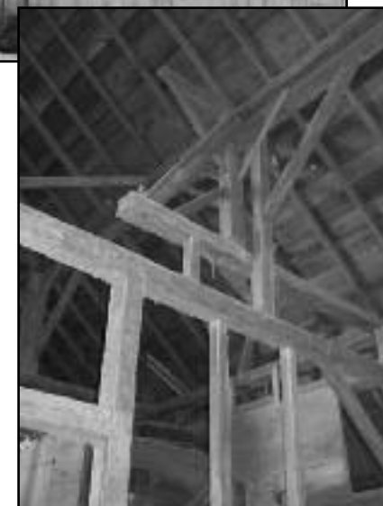
Above left: Dovetail notching alongside mortise and tenon joinery in the Poorman barn. Right: Tie beam cut to accommodate the hay rack receives reinforcement from double framing. So far no cables or creative carpentry have been employed to compensate for this excision of the structurally significant tie beam.
