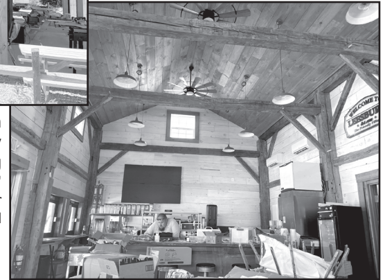
Exposed timber framing on the inside of the "new dairy barn" and outdoor seating in the "barnyard."
