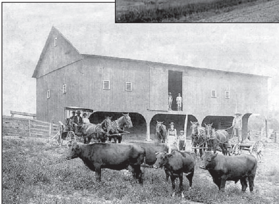
Left: The old Kornmiller barn (circa 1887-1895), a Pennsylvania German bank barn with a posted forebay in Hocking County. Ohio cultural geographer, Dr. Hubert G.H. Wilhelm, identified State Route 180 in Hocking County as the southern limit of the occurrence of the Pennsylvania German barn in Ohio. This barn burned to the ground after being struck by lightning in 1970.
