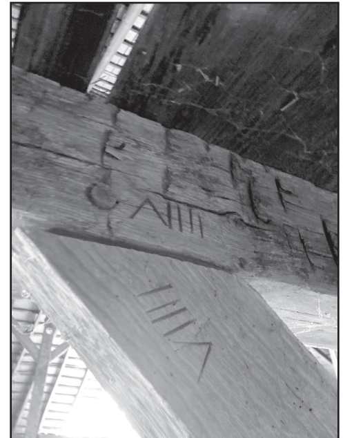
Brace connecting to tie beam with marriage marks at joint 9 (VIII). Presumably the 4 had an odd use of Roman numerals to prevent confusion between IV and VI and — 4 and 6. Similarly the 9 could get confused with an 11 — IX and XI.
