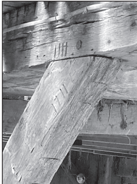
Brace connecting to tie beam with marriage marks at joint 4 (IIII).
