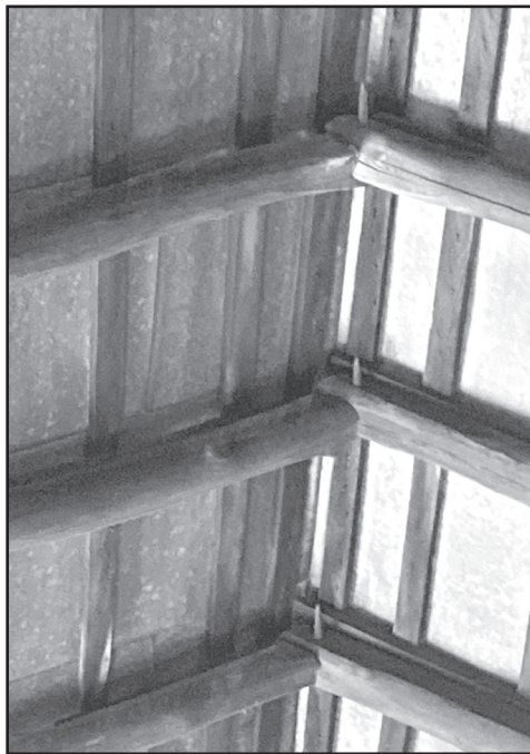
The barn has no ridge pole. The rafters are pinned together with wooden pegs.
