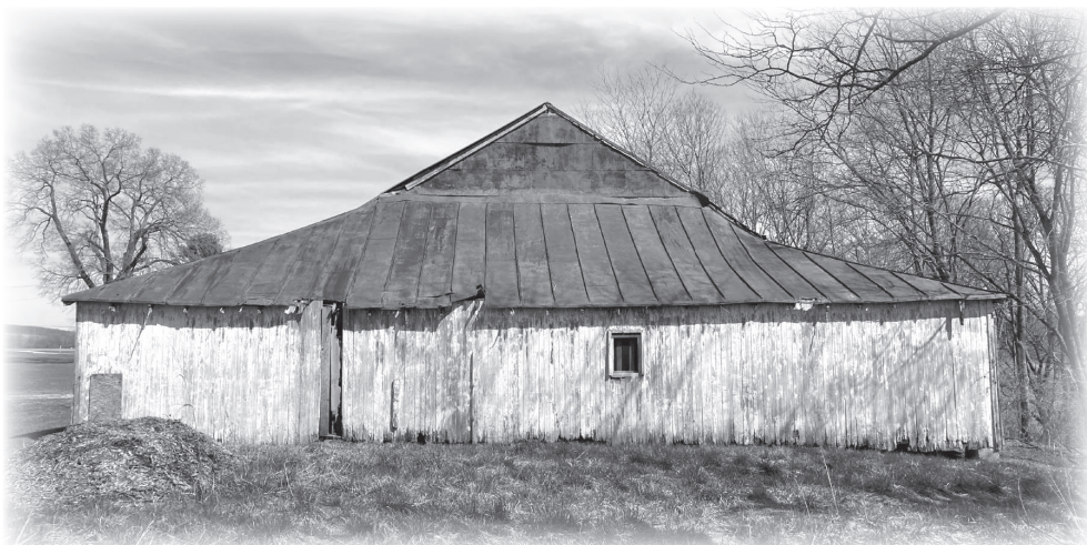
Rear view of Hopewell barn with side and rear additions. Gable roof defines the dimensions of the original hand hewn structure.
