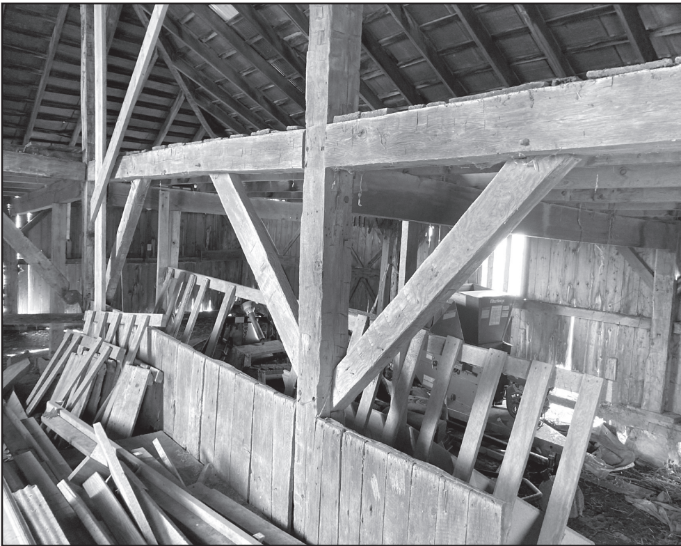
This image shows the 4 foot layout on the bracing, remnants of the waste wall, boards added for temporary stability, and a view into a side and rear addition.
