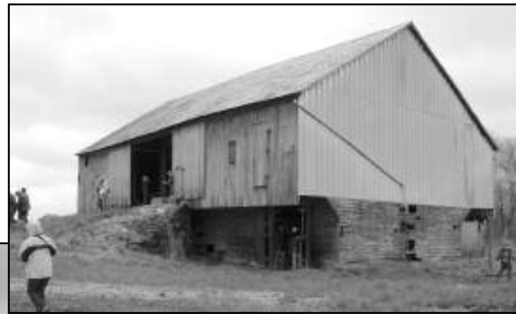
Left: Miller barn with double overhang and ramp up to the threshing floor. Above: Interesting joinery in the Miller barn basement.
