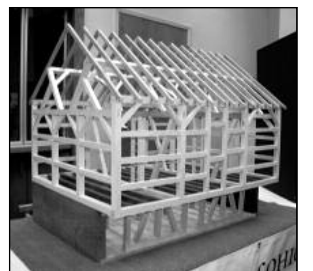
Model Pennsylvania bank barn with forebay used in the JBD session at the Ohio Barn Conference.
