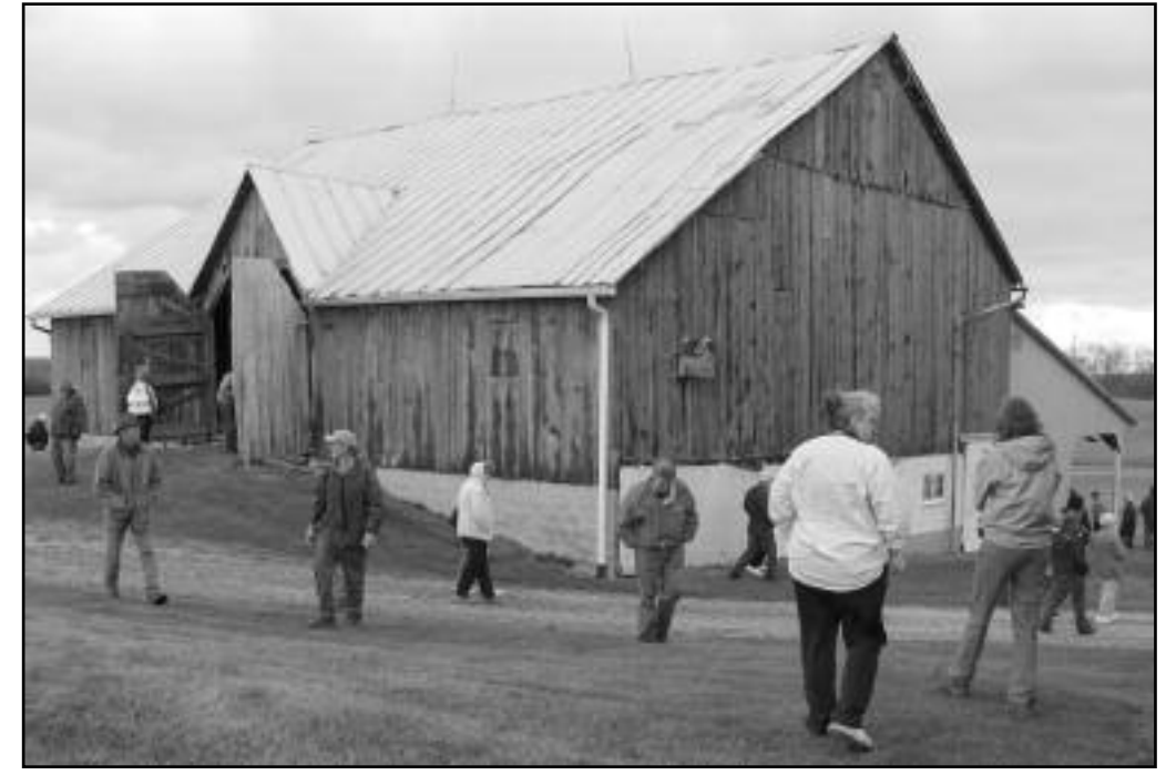
Above: The overhanging forebay on the upper side of the Mertz barn has recently been closed in with a cement block foundation.
