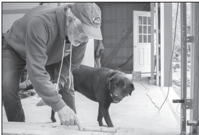
Dan Troth, a contractor who rebuilds timber structures and vice president of Friends of Ohio Barns, points to layout marks on a post made by a historic barn's original builders, while dog Layla looks on.
