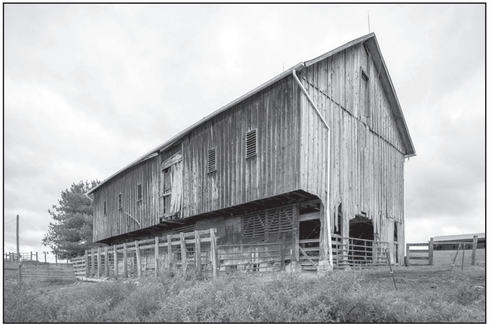
Overhanging forebay of a classic Pennsylvania German barn. Note wind doors and louvered vents on the level of the threshing floor and basement for livestock.
