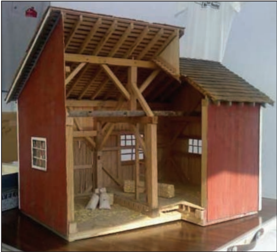
Model timber frame structure built by Lowell Finley.
