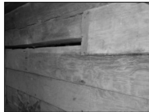
Remnant siding made of hand riven clapboards from Ohio's primeval trees still cover the old hand-hewn timbers in Gene Carter's double crib log barn.
