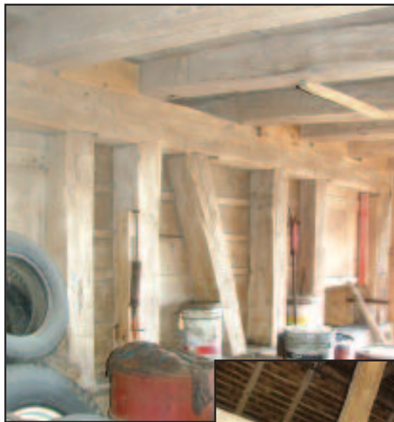
Above: Basement wall with hefty supports and floor joists. Right: A bow string truss.
