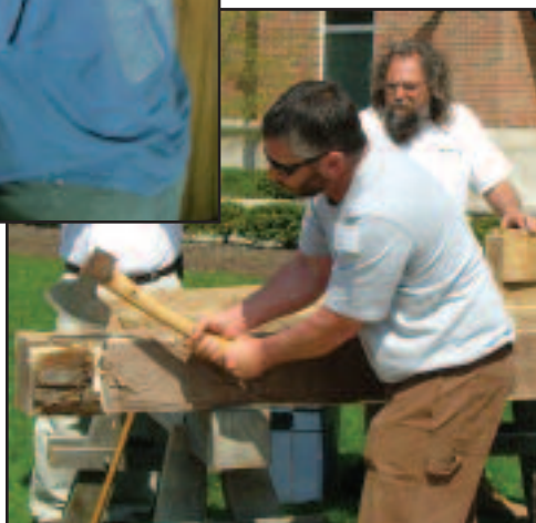
Left: Brian demonstrates the technique of using an adze. Above: Tom inspects the seaming of a rafter plate. Right: Brian demonstrates use of a broadaxe.
