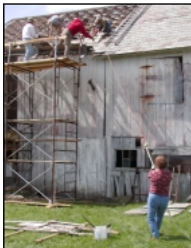
Susan Ramser of Danville lowers slate from the roof with a rope and a sling.
