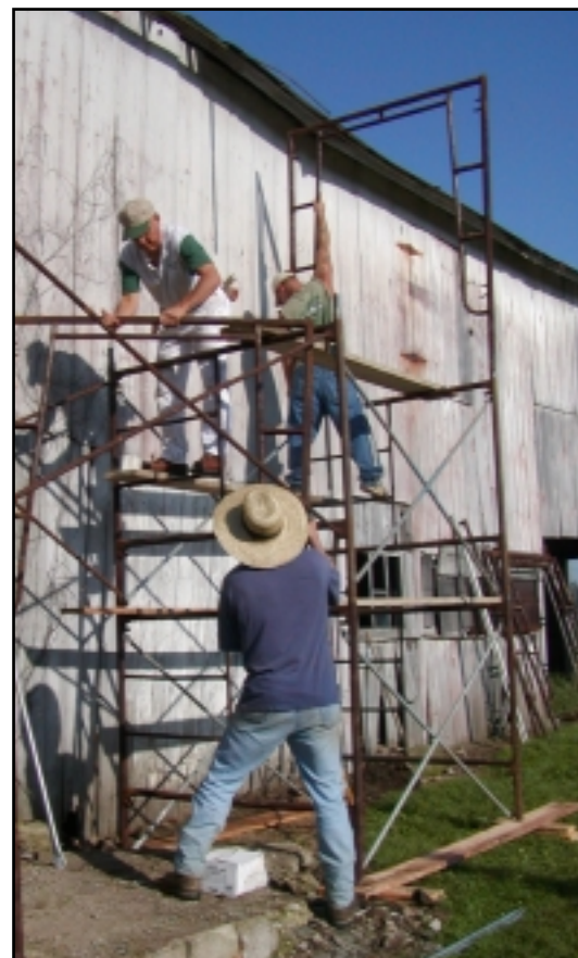
Above: Putting up scaffolding was the first lesson of the day. Having the right equipment for the job is essential.
