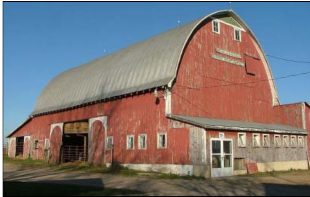
This dairy barn, located in Salem Township, Champaign County, is a bow-roof, side drive, Yankee hay barn with numerous additional sheds. The decorative painted arches and trim are typical of turn of the century barns on the Indiana/Ohio border.
