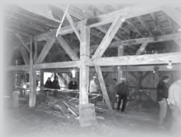
Right: Framing above the third floor is still open for interpretation. It may be that the trusses were used for support to enable the teams and wagon to turn around inside the barn and exit going forward instead of having the horses back out across the bridge with the wagons still attached.
