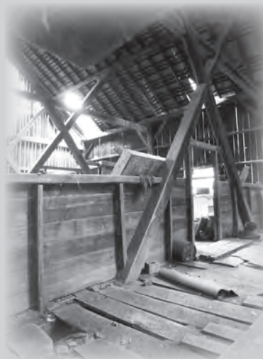
Left: Portions of two central bents and one end wall. Note the rear of the waste wall (used to keep grains within the threshing floor area for collection) running across the mid-height of the image. A doorway has been cut into the waste wall.
