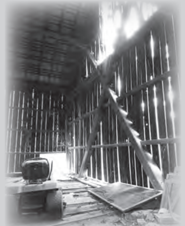
Right: The bent on end wall of the barn with timbers extending from the floor to the purlins.
