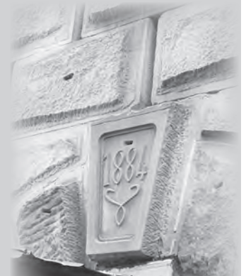
Above: The keystone in the arch over the basement entry with an image of the stone grapple used to lift the stones into place. Every stone, including the keystone, have a centrally located hole for the stone grapple.
