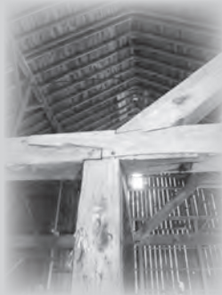
Left: A little extra support in the framing used in the Brown-Bender barn.
